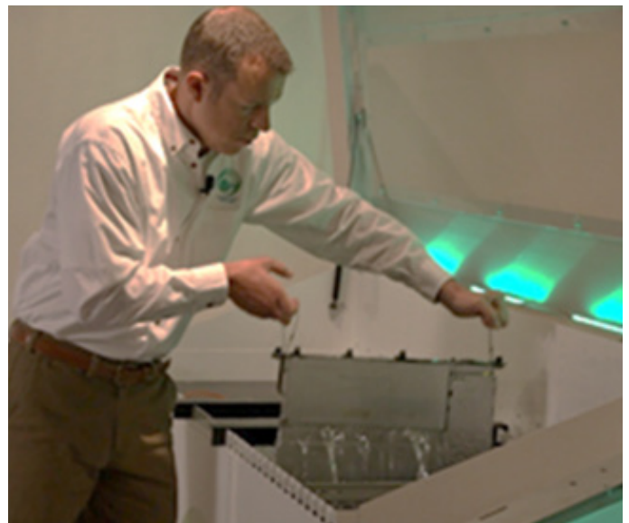
Figure 1. A Server Board is Removed from a Container of Mineral Oil that Provides Cooling of the Hot Running Server Electronics [3]
