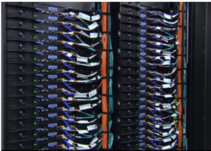
Figure 2. The Cooling System for the SuperMUC Computer Uses Hot-Water Technology to Cool 150,000 Cores [5]
